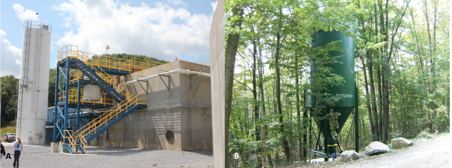
A) This is an example of a large water treatment facility. This facility cost $14.4 million, and requires a full time employ to maintain. B) A “lime doser” is really just a silo filled with basic chemicals that regulates how much of this chemical is added at a time.
