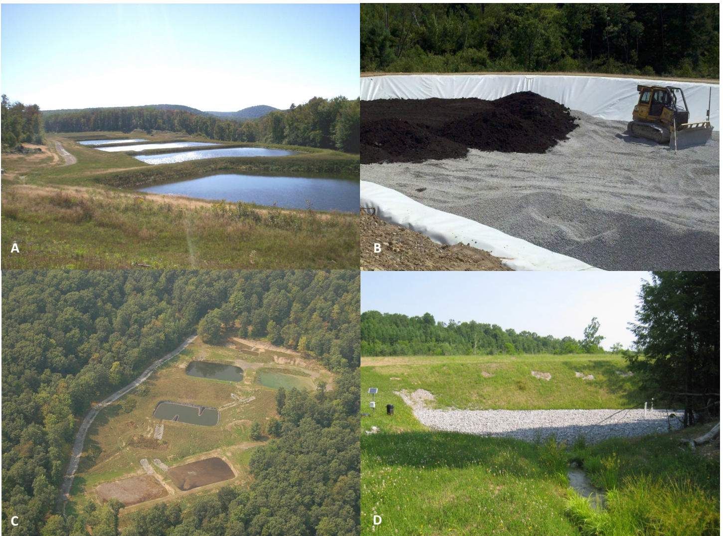
A) Large treatment systems like this one contain multiple “cells” which treat water. If one of them is damaged or needs work, water can be diverted to the other cells allowing treatment to continue. B) In this system pipes are placed at the bottom of the pond, with limestone over top. Mushroom compost is placed on top of to promote bacterial growth. Water must flow vertically through all the layers to the pipes on the bottom, so these types of systems are called vertical flow ponds. C) Systems are often times quite large and utilize multiple types of treatment . D) This type of passive treatment is call a limestone cell and raises the pH of water.
